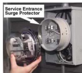
Figure 3. A surge arrester installed on the electric meter service entrance. Other arresters installed inside near the main panel can also protect phone and cable lines.
